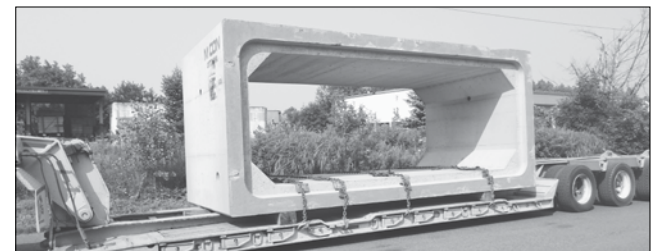
Submitted One section of the new concrete culvert sits on a flatbed trailer, awaiting installation by a giant crane.
