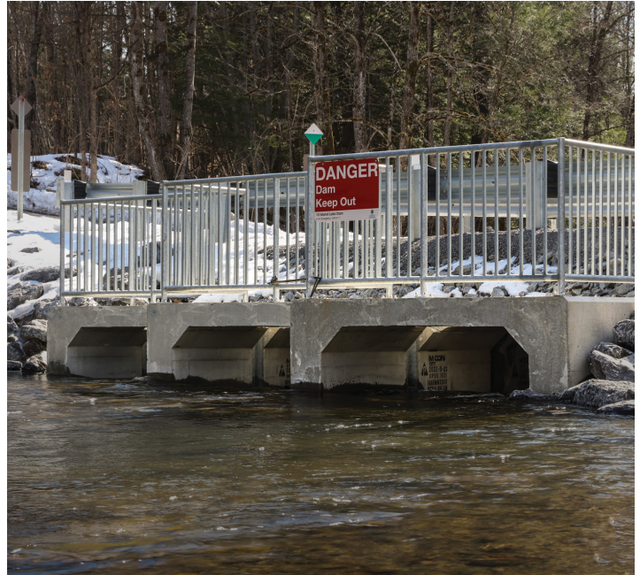
Completed box culvert dam structure.
