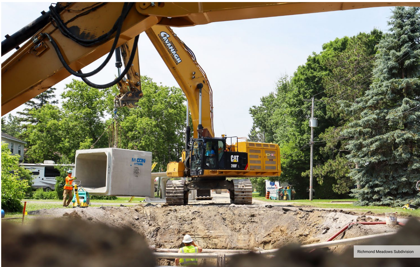
Ottawa Hospital Civic Campus Parking Garage Retaining Walls
